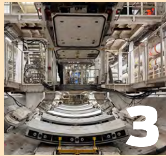
[ABOVE]: ■ The TBM operator monitors all operations from the control room. ■ Multi-service vehicles are used to transport the tunnel segments to the TBM. ■ The segment feeder brings in tunnel segments as the vacuum erector awaits overhead, preparing to move each segment into place. ■ The TBM has 54 hydraulic thrust cylinders that push against the tunnel ring to move the TBM forward.
