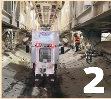
[ABOVE]: ■ The TBM operator monitors all operations from the control room. ■ Multi-service vehicles are used to transport the tunnel segments to the TBM. ■ The segment feeder brings in tunnel segments as the vacuum erector awaits overhead, preparing to move each segment into place. ■ The TBM has 54 hydraulic thrust cylinders that push against the tunnel ring to move the TBM forward.
