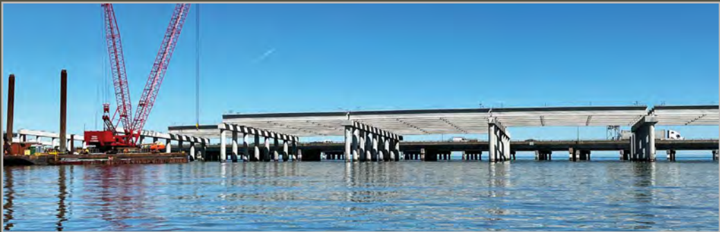
A view from the water of the piles, caps and girders for South Trestle bridge.
