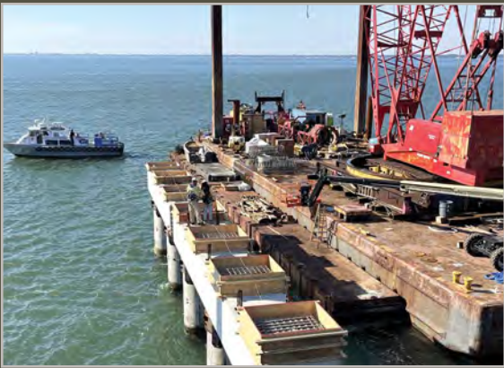
Crews work to prepare the pile caps to receive their bearing pedestals.
