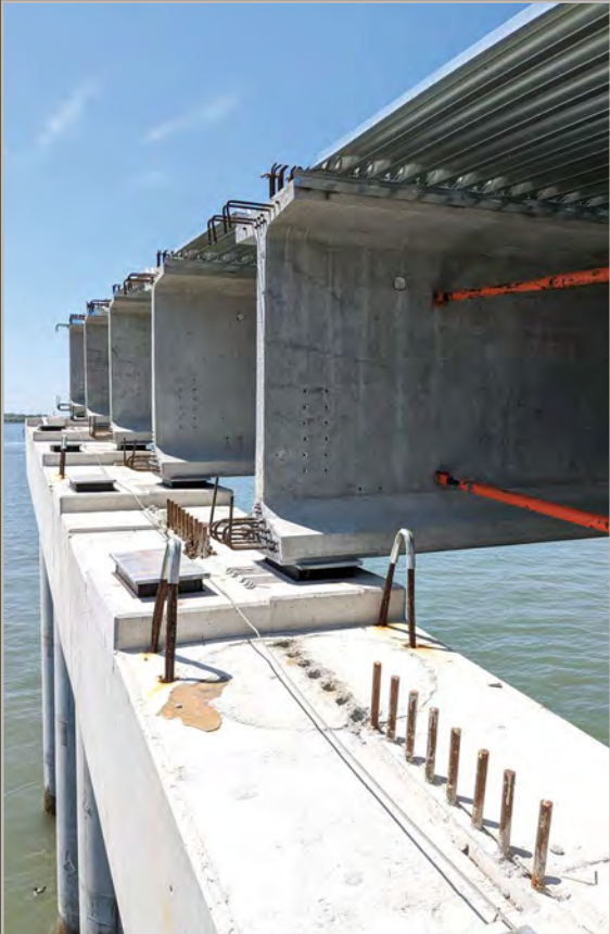
85" concrete girders land on each pier cap with elastomeric bearings carrying the immense load.
