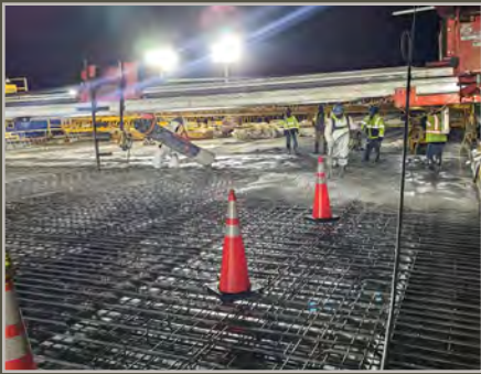
Specialized equipment is used to ensure bridge deck concrete is precisely placed and leveled.
