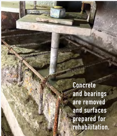
Beam ends are prepared and reinforcement receives a special coating to prevent future corrosion.
