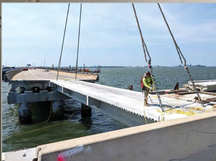
Crews carefully remove segments of the old bridges, which will be treated and used in existing artificial reefs in partnership with the Virginia Marine Resources Commission.
