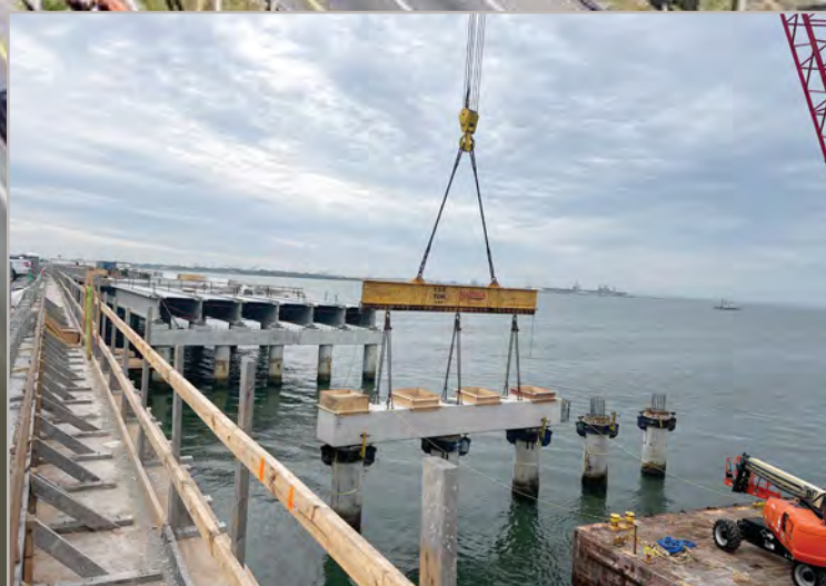
Caps are installed on top of the piles to support the girders.
