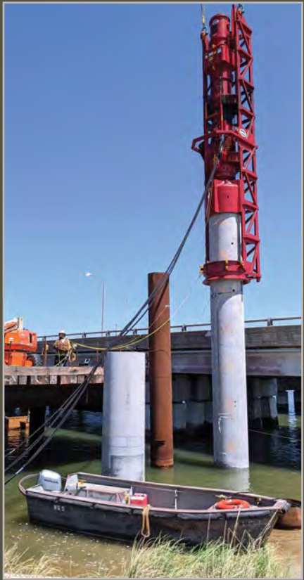
New piles are driven deep into the seabed to provide support for the new bridges.
