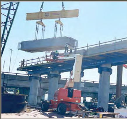
A crane is utilized to move the pile cap into place on top of the piles.
