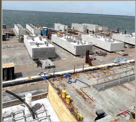
Pile caps are staged for placement.
