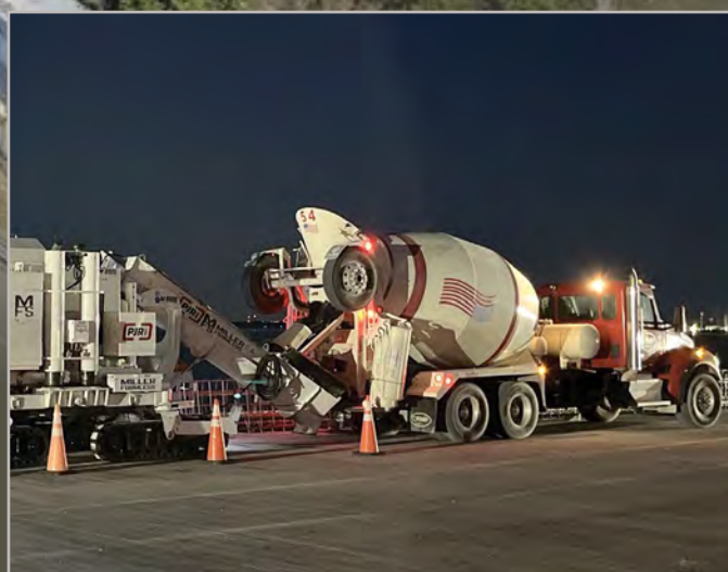
Concrete trucks deliver material to build parapet walls on new and widened structures.
