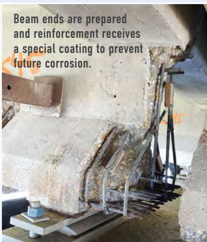
Concrete and bearings are removed and surfaces prepared for rehabilitation.
