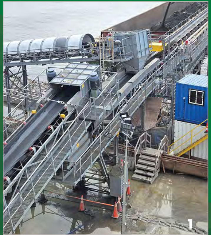
[1] Spoils excavated by the TBM are transported by conveyor belt to an awaiting barge.
